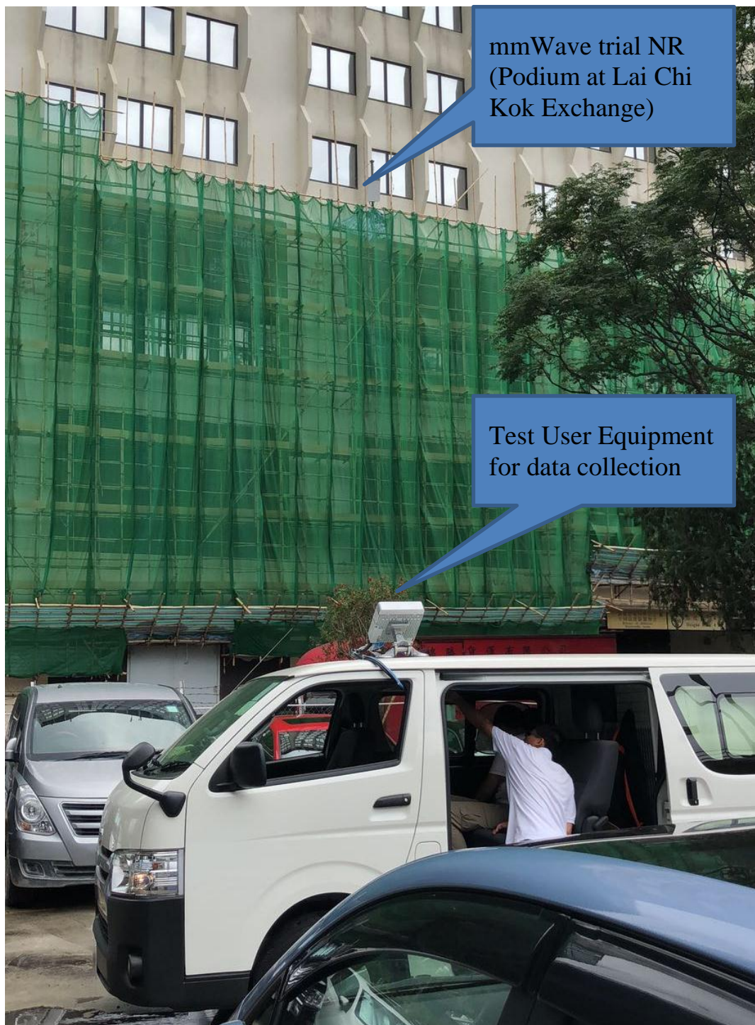
Figure : Antenna mounting viewed from the street
