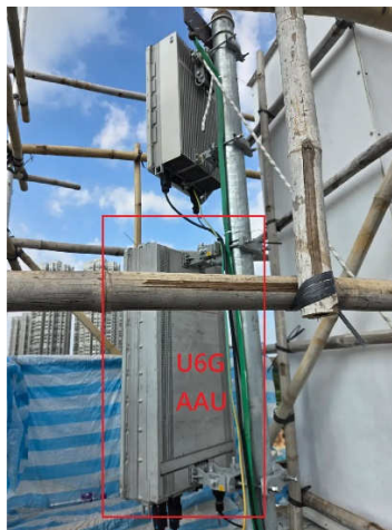
Figure 1. U6G AAU Installation Set Up
